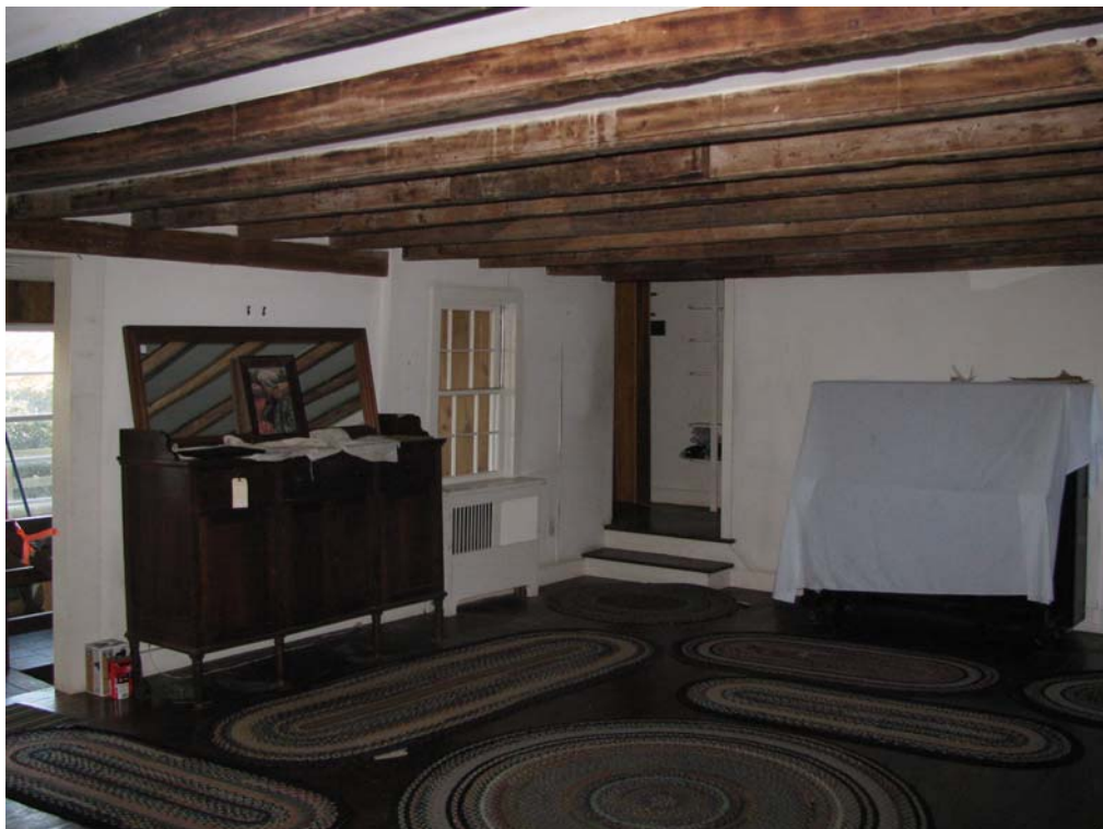
Exposed Beams in Family Room
