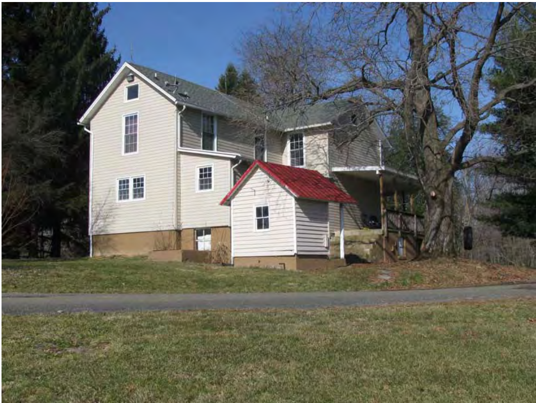
House Number 1 (Rear View)
